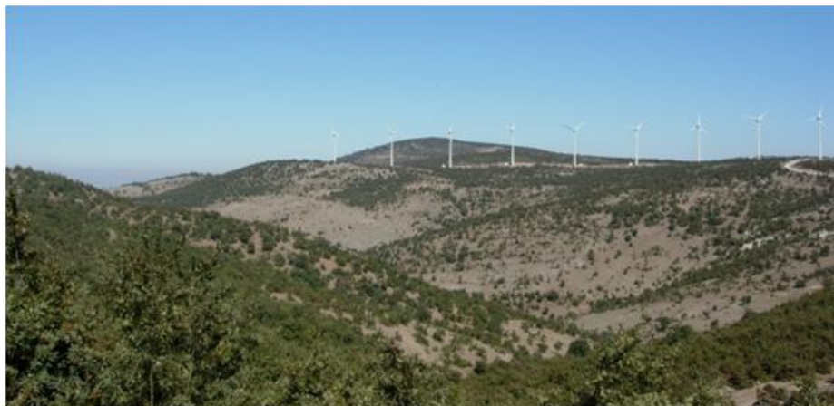
Figure 1-2: View of the existing plant
