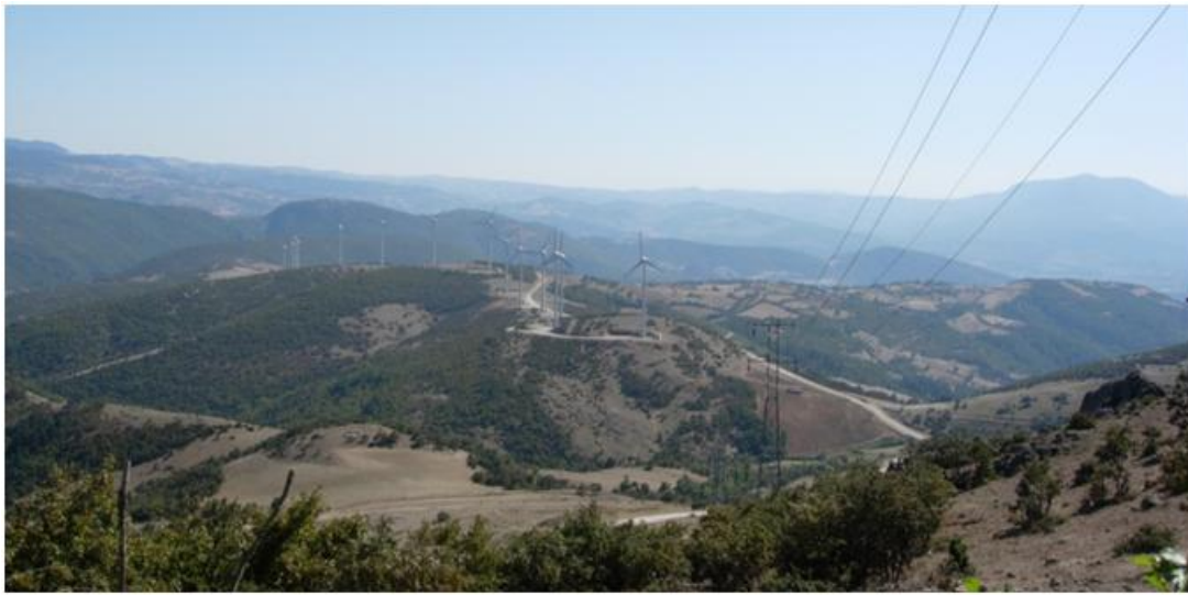
Figure 1-1: View of the existing plant
