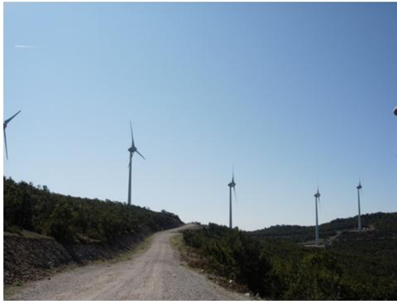
Figure 1-3: View of the existing plant
