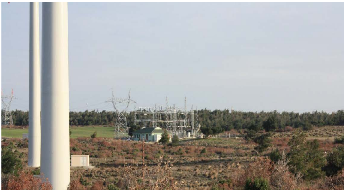
Figure 1-3: Existing switchyard at the Çamseki WWP
